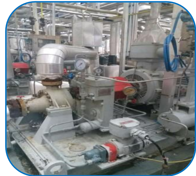
▲ Fujian United Petrochemical Co., Ltd 2000-P40412AR/BR Propylene Product Pump GSB-Q5-171/580 Power: 255KW
